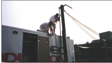
Figure 2.96 Cables often have to be off the ground because they can cause accidental falls or be run over, or simply because the local officials say so. So they may be "flown" as they leave the truck. (Source: Tim Stoffel)
